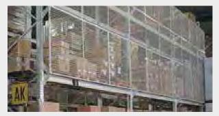
Anti collapse mesh prevents any risk of spillage from pallets, offering protection for a variety of scenarios.
