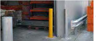
Metal safety bollards are available either painted or galvanised. Manufactured from robust steel tube, these 164mm diameter barriers are available in a range of heights.
